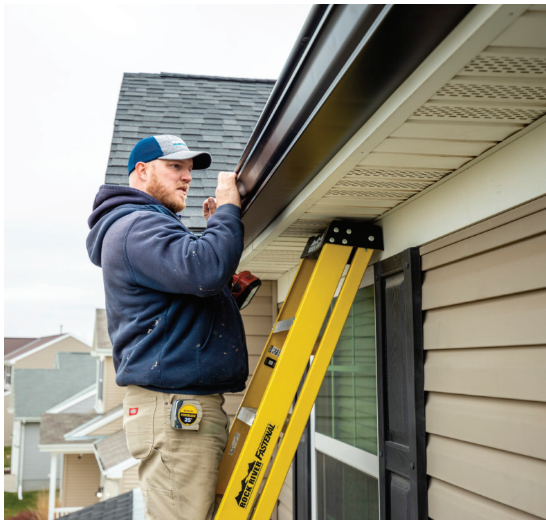
Photo courtesy of Thrasher Foundation Repair
